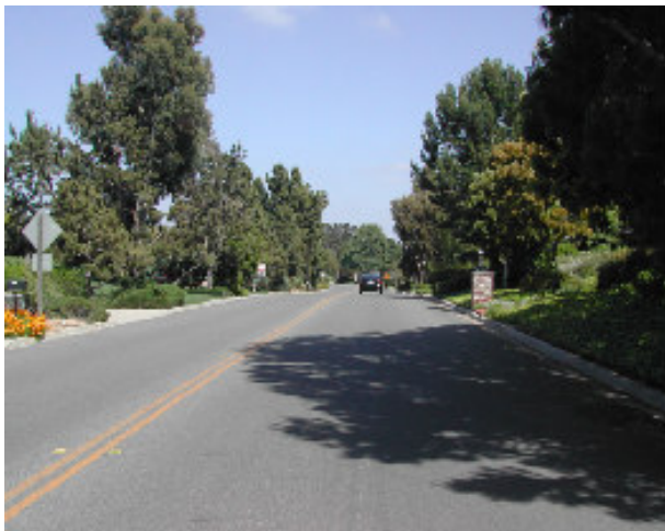
Highland Drive is classified as a collector road. The road is 40' wide, with curb and gutter.
