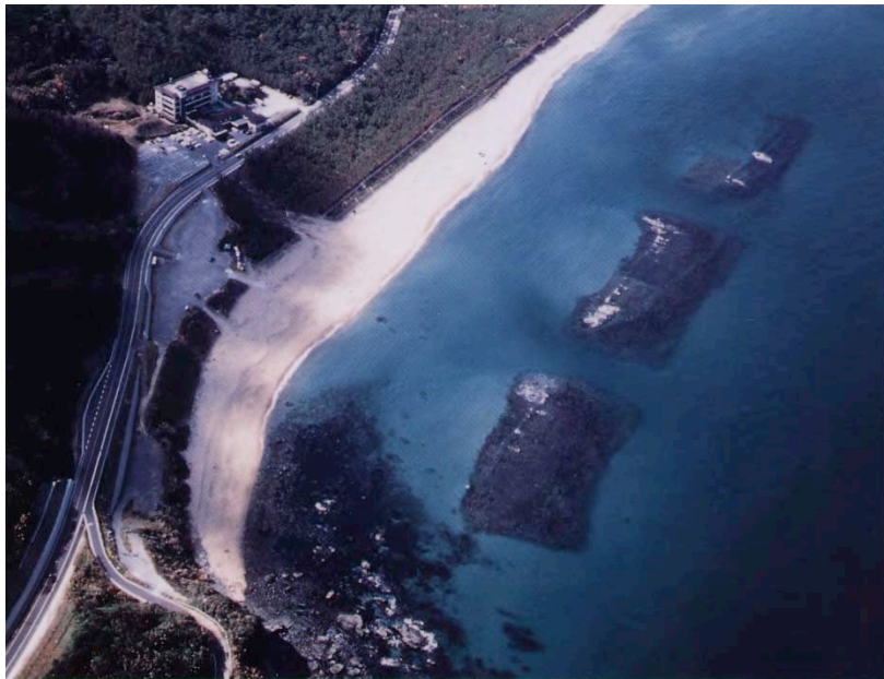
Figure 4.1. Submerged reefs for coastal protection in Japan
