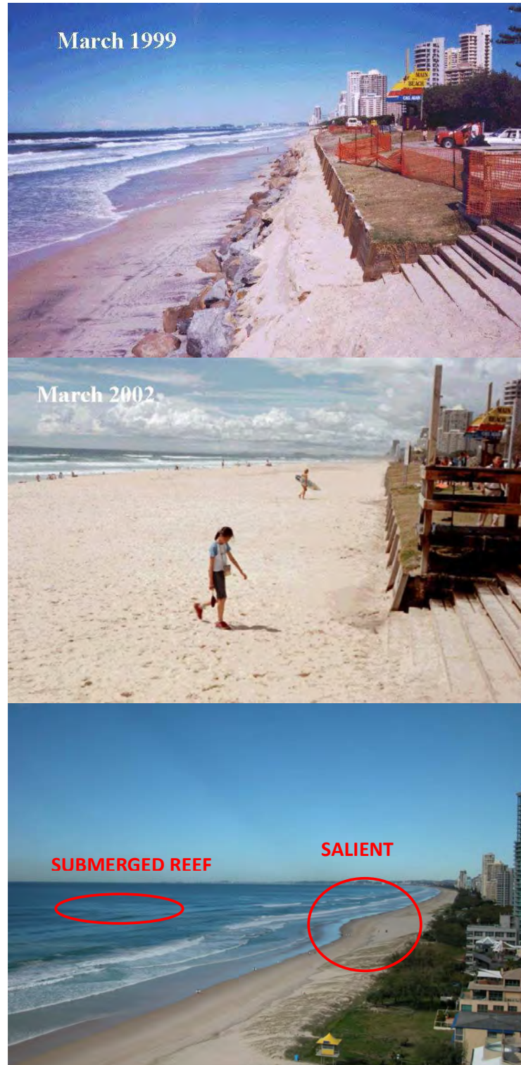
Figure 5. Coastal protection with the Narrowneck submerged reef. Top to Bottom: Beach condition before reef construction (construction commenced in August 1999); After reef construction; The view looking south showing the wide salient in the lee of the reef.
