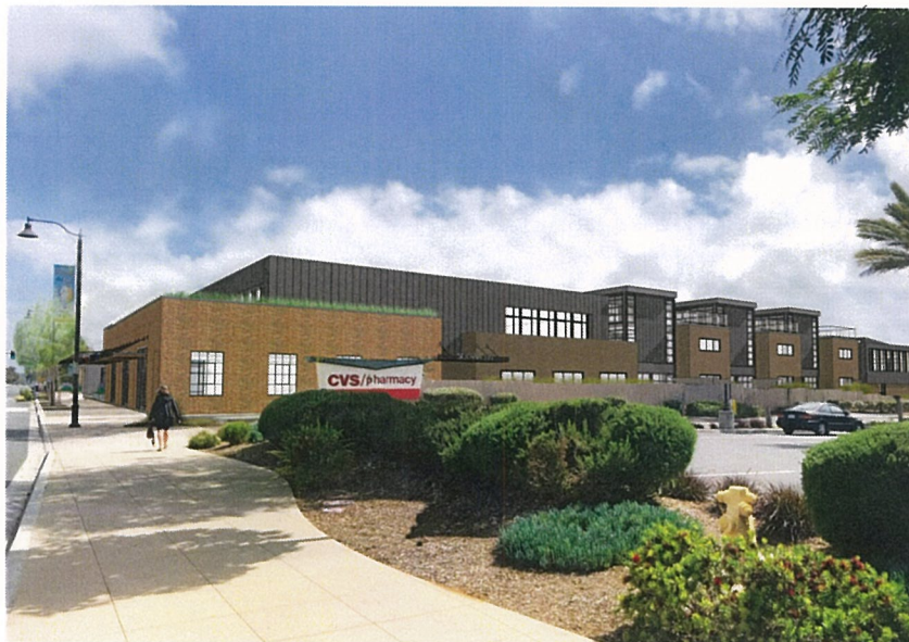
2 ENTITLED OFFICE NORTH FROM CVS (NORTHEAST CORNER)
