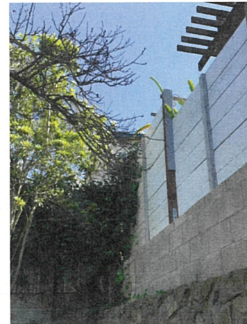
6. VIEW TO SOUTH EAST FROM REAR YARD
