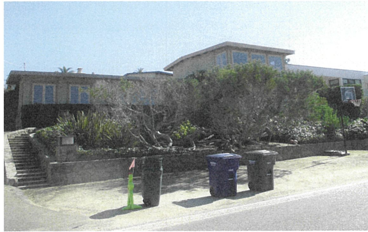
2. VIEW TO EAST FROM FRONT OF HOUSE
