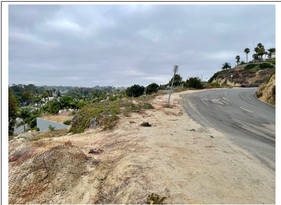
Photo Point 2. View to the north at entry to site along Highland Drive. July 8, 2022.
