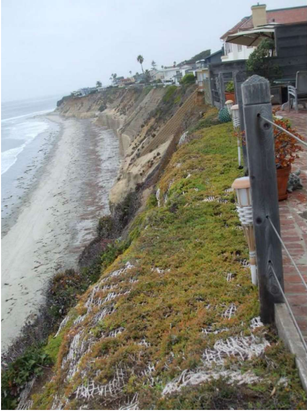
Photo 29: 309 Pacific Avenue looking north (November 4, 2013).
