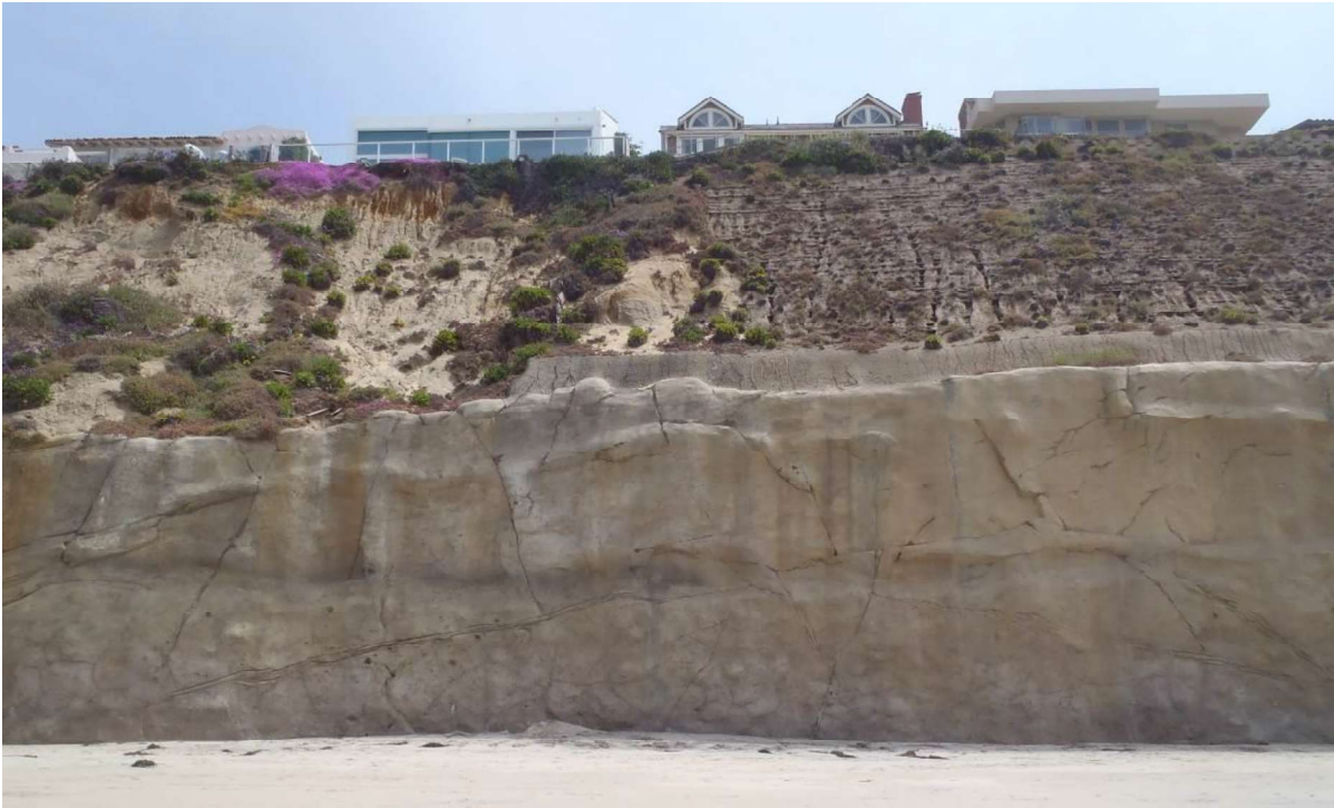
Photo 4: Seawall below 301 to 261 Pacific Avenue (April 26, 2023).
