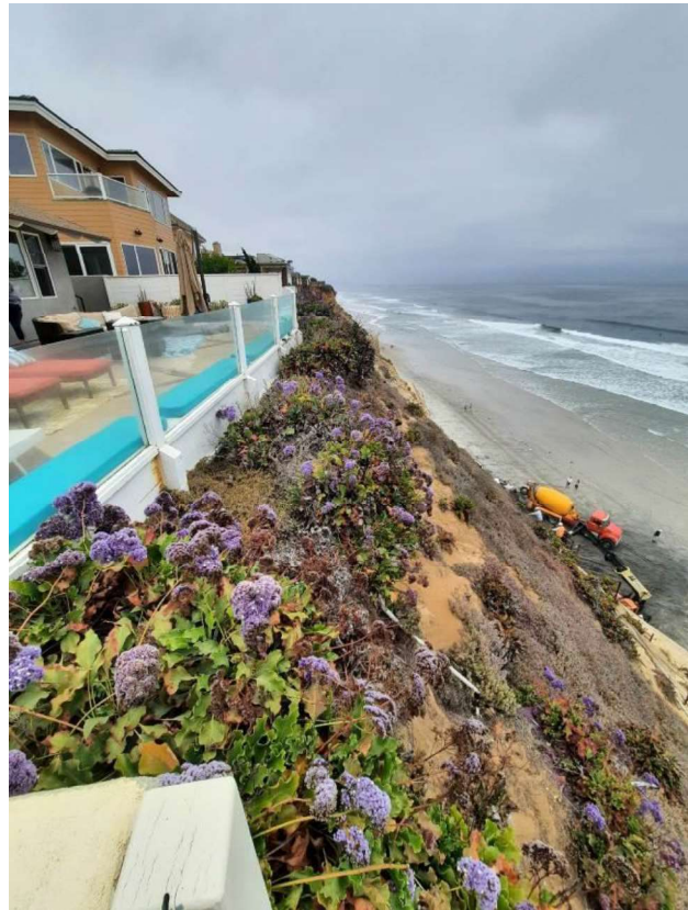
Photo 18: 249 Pacific Avenue looking south (May 19, 2022).
