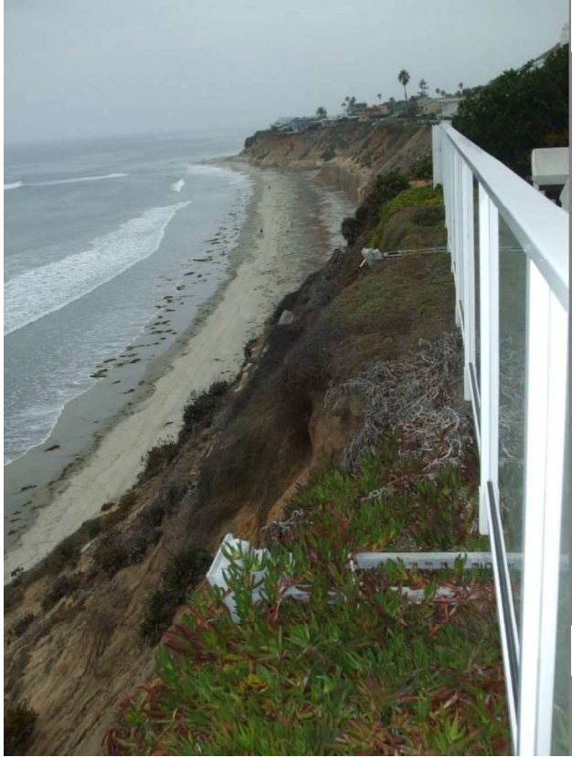
Photo 25: 269 Pacific Avenue looking north (November 4, 2013).
