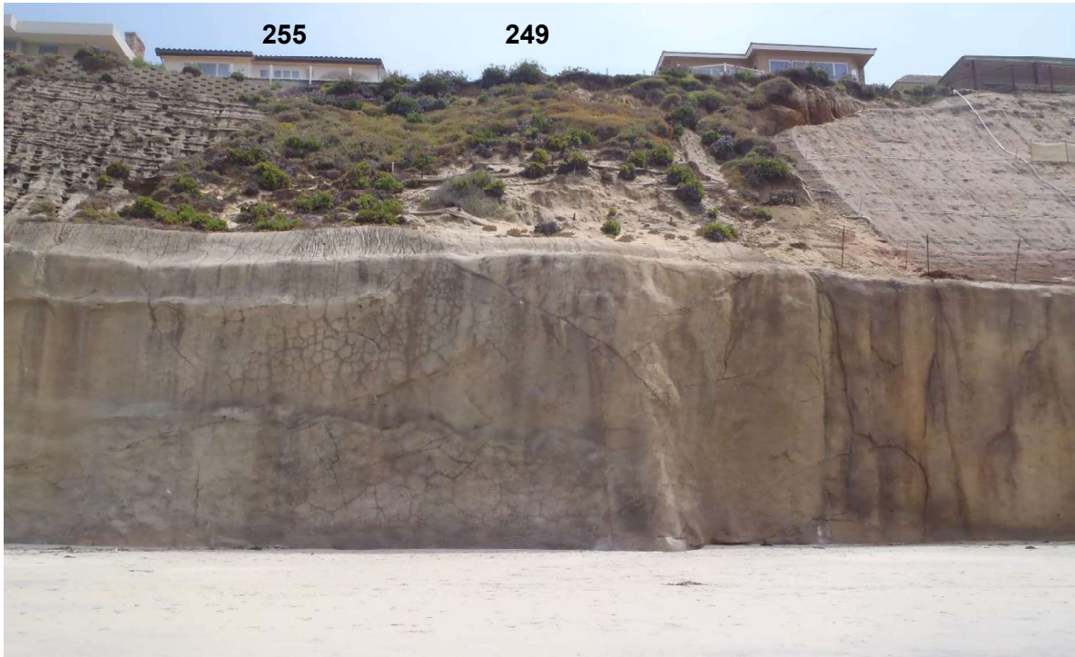
Photo 6: Seawall below 255 to 249 Pacific Avenue (April 26, 2023)
