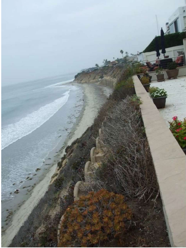
Photo 21: 261 Pacific Avenue looking north (November 4, 2013).
