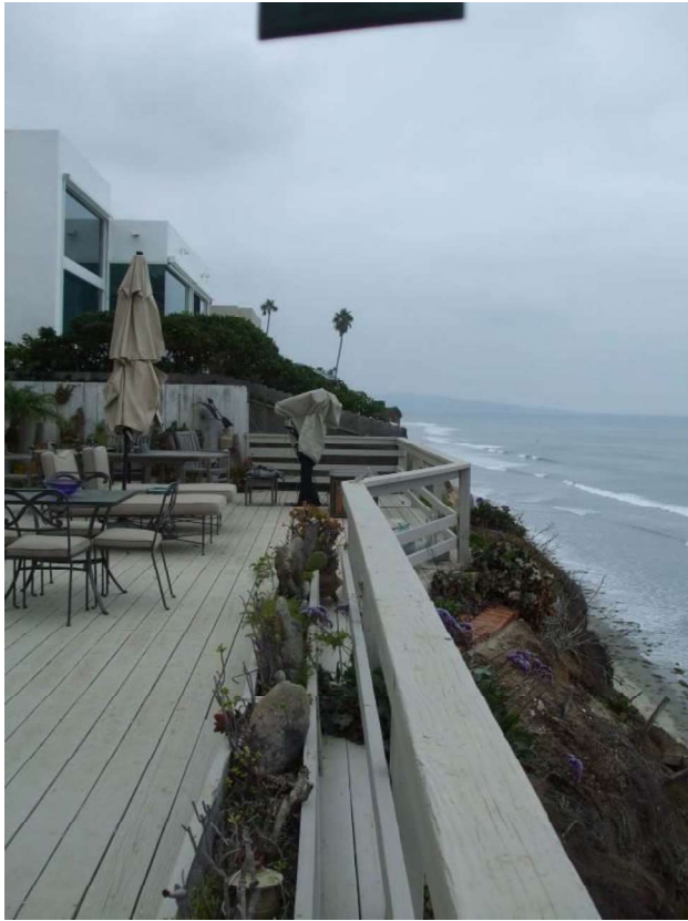
Photo 27: 301 Pacific Avenue looking south (November 4, 2013).
