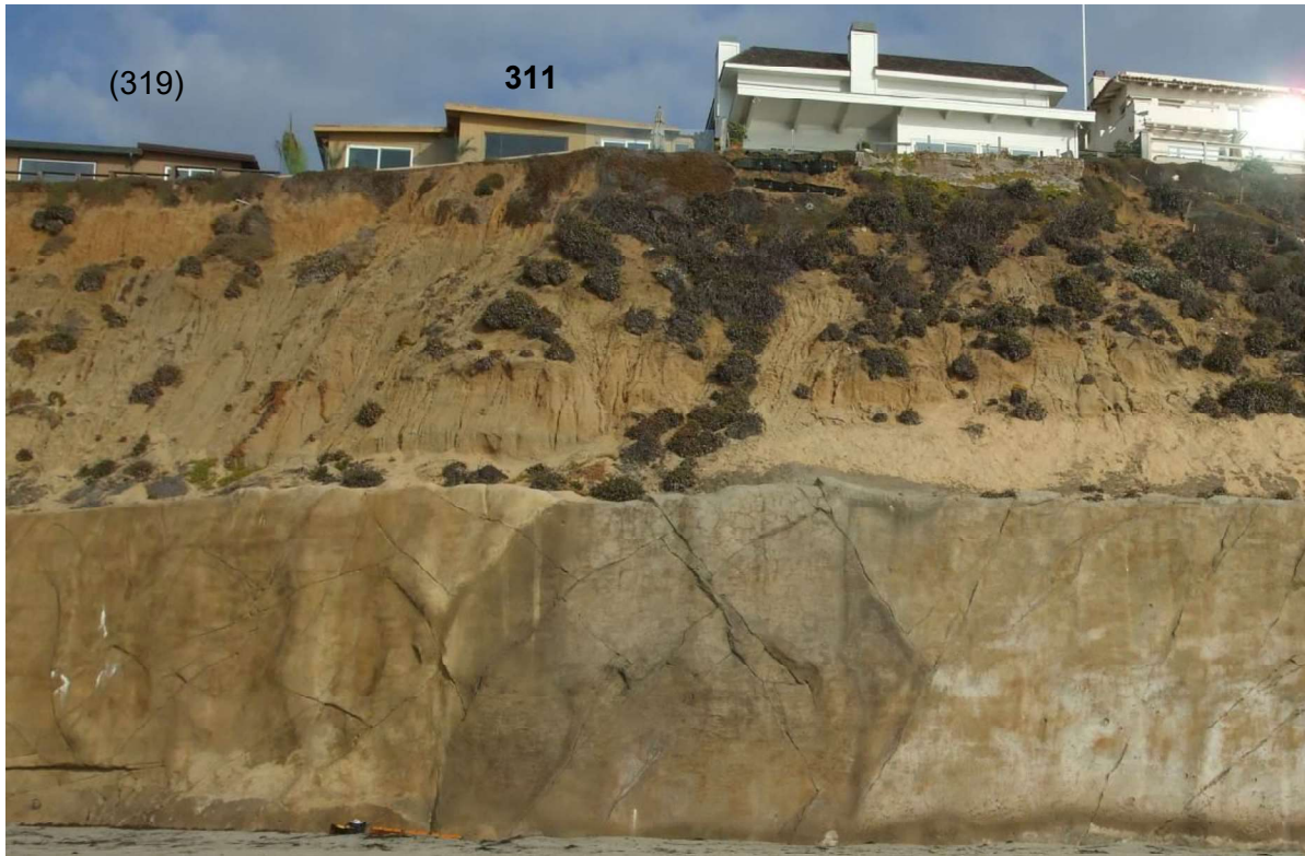
Photo 7: Upper bluff below 311 to 309 Pacific Avenue (November 4, 2013).
