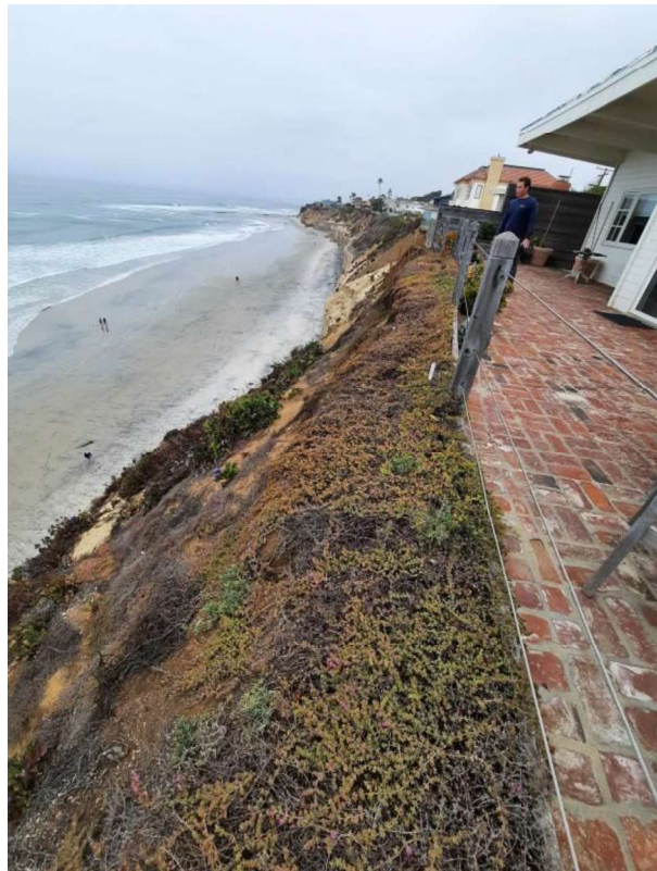
Photo 30: 309 Pacific Avenue looking north (May 19, 2022).
