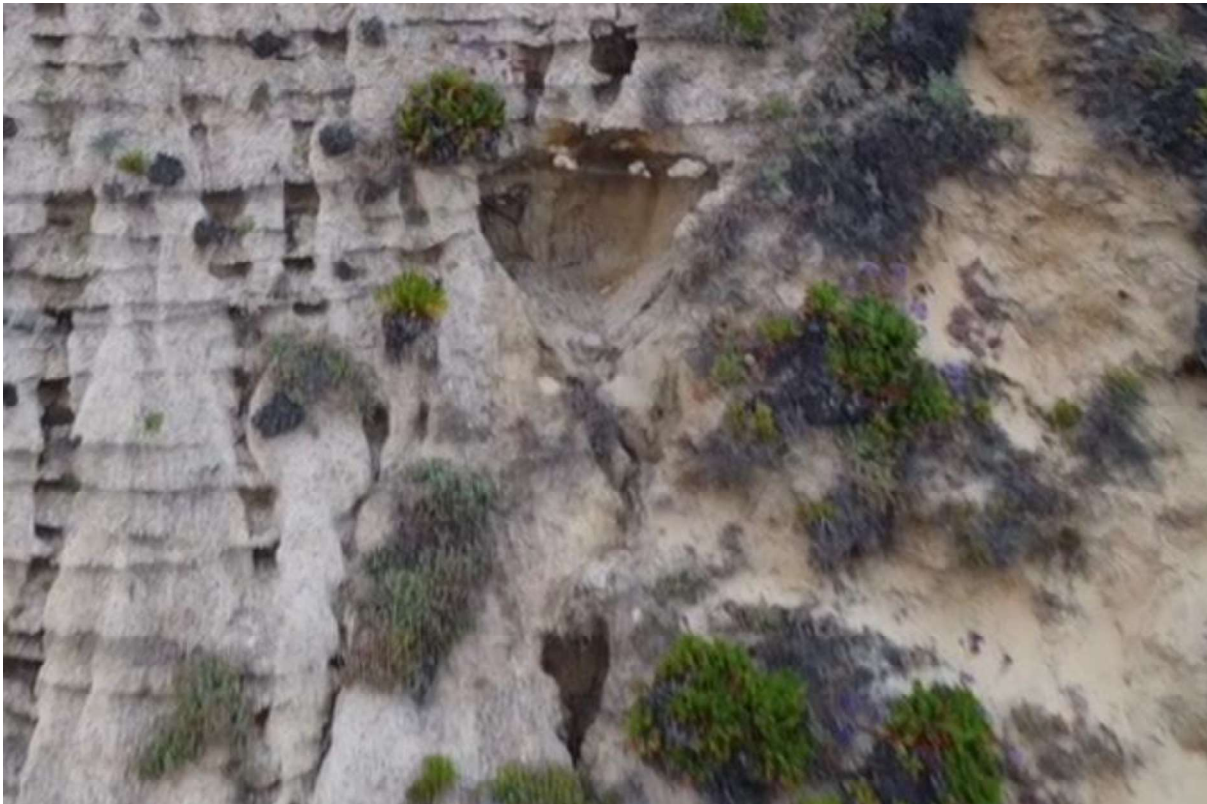
Photo 14: Screen shot of large and small erosion gullies below 255 Pacific Avenue provided by property owner drone footage (July 19, 2023).
