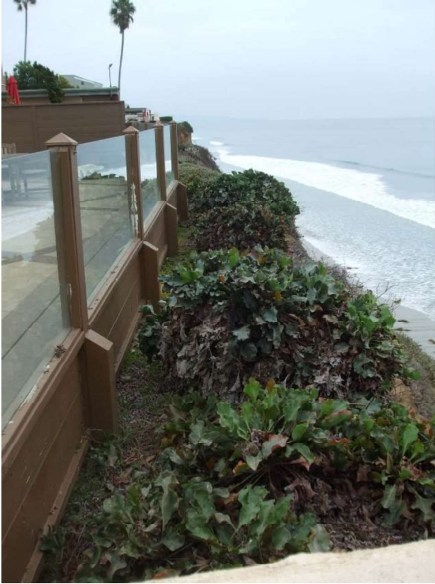
Photo 17: 249 Pacific Avenue looking south (November 4, 2013).
