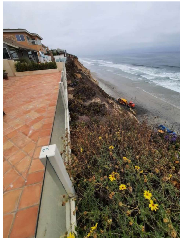
Photo 20: 255 Pacific Avenue looking south (May 19, 2022).
