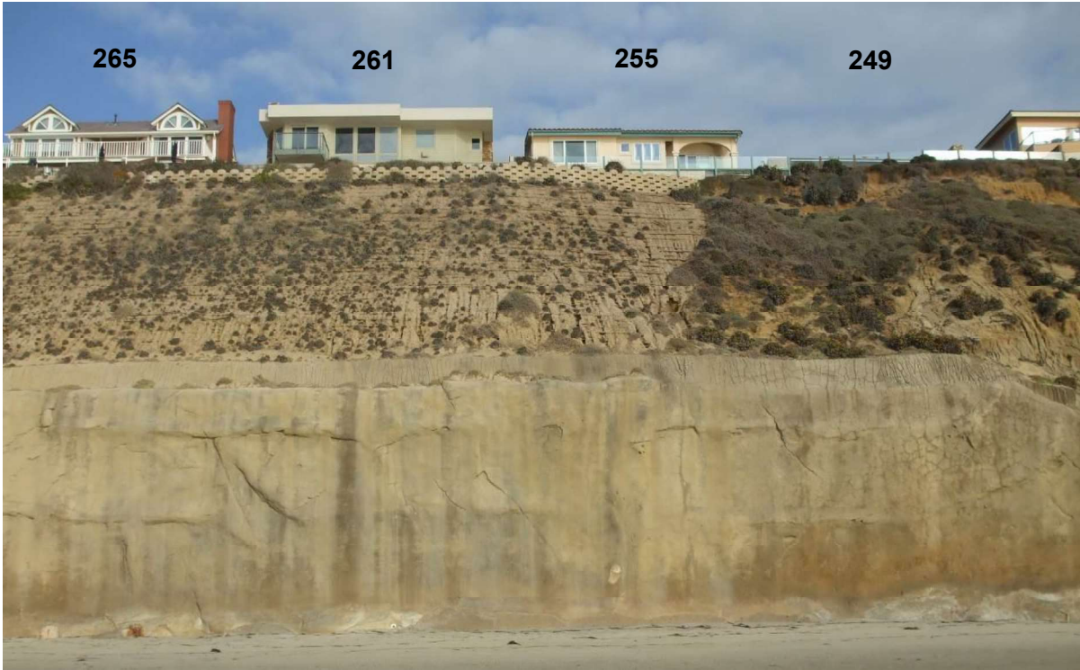
Photo 11: Upper bluff below 265 to 249 Pacific Avenue (November 4, 2013).
